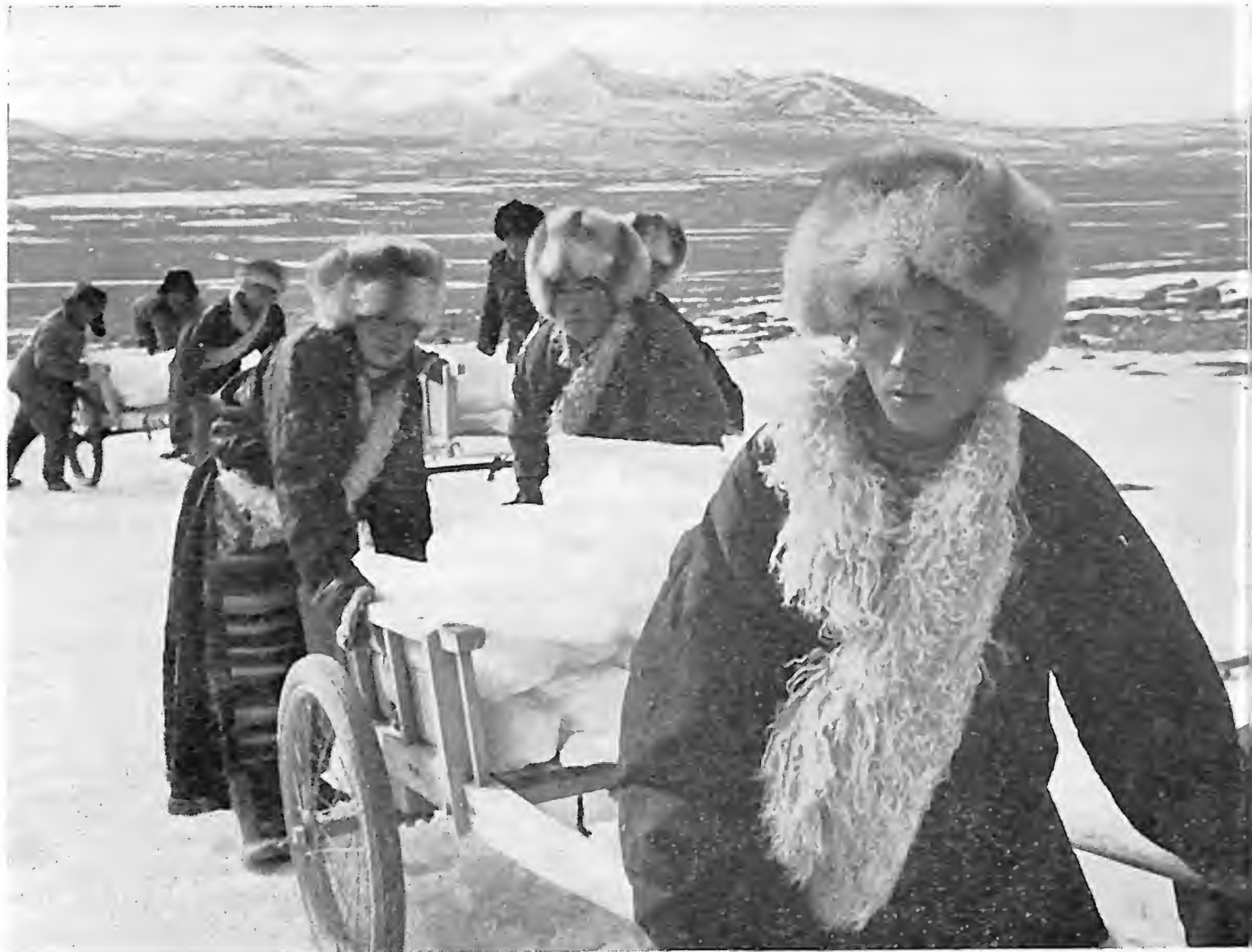
Clearing ice from the highway.
